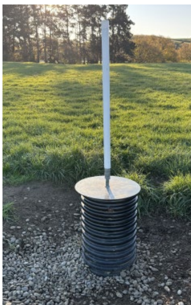
Figure 9. A vertical sump system is used so the water from a depression can drain to the ditch at the edge of the paddock.
