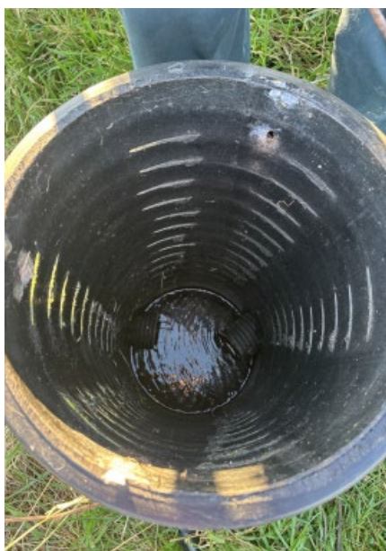
Figure 9. A vertical sump system is used so the water from a depression can drain to the ditch at the edge of the paddock.
