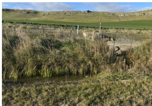
Figure 27. An interception drain catches runoff from a hard surface before it can scour part of the paddock (before and after).
